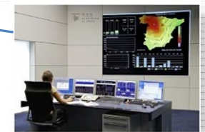
Control Center for Renewable Energies
