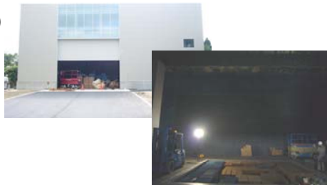
Under construction (2010.10E) (Uji campus, Kyoto Univ.)
